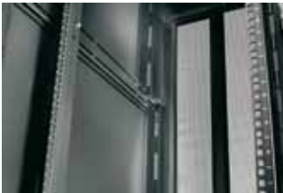
19 inch rear risers divided into three sections
